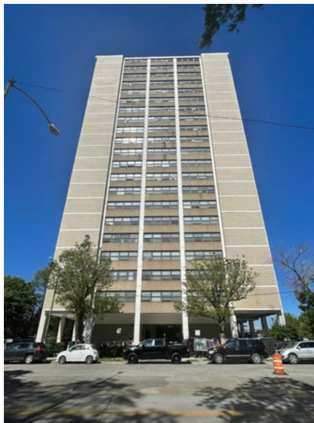
Image: Courtesy of Preservation of Affordable Housing Inc. Island Terrace, a 22-story affordable housing development located in Chicago's Woodlawn neighborhood that was built in 1969, is undergoing renovations thanks to 9% and 4% low-income housing tax credits.
