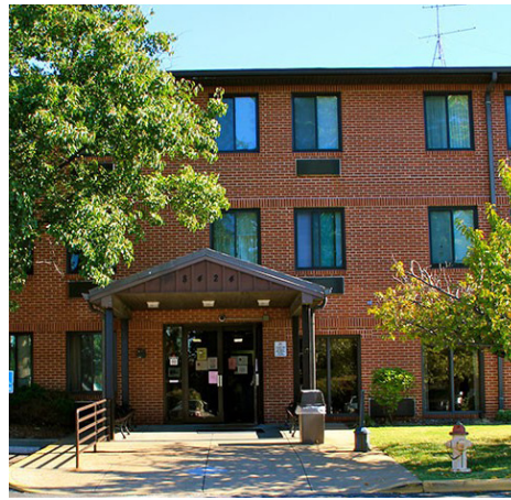
St. John Neumann Apartments—Jennings
