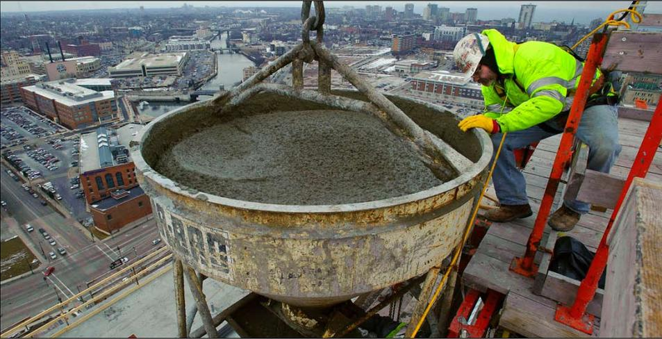
*A worker positions a concrete bucket while pouring the mechanical penthouse over the 30th floor of the Moderne.*
