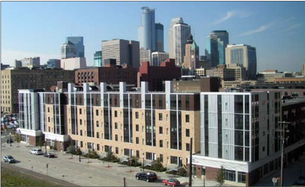
St. Anthony Mills Apartments, Minneapolis
