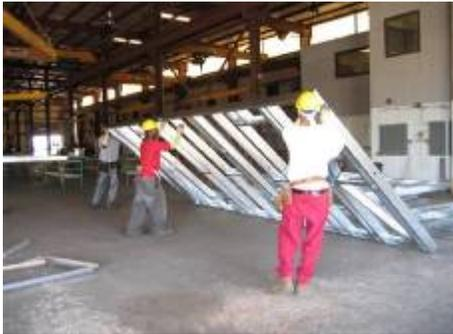
Workers erect a steel-frame panel at the Housing International Gulf Coast, Inc. panelized housing facility in Reserve, LA.
